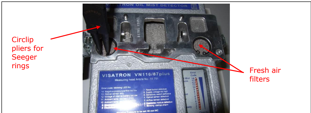
Figure 45: Exchange of the air filters
